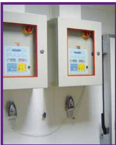
Controllo temperatura in celle frigo
