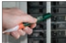
Non-contact InfraRed Temperature measurement
